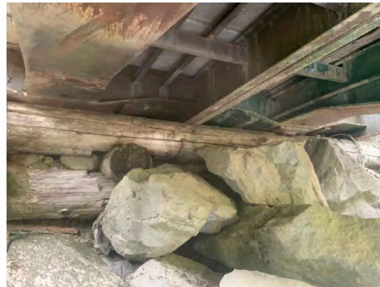
Right Bank Abutment when facing downstream
