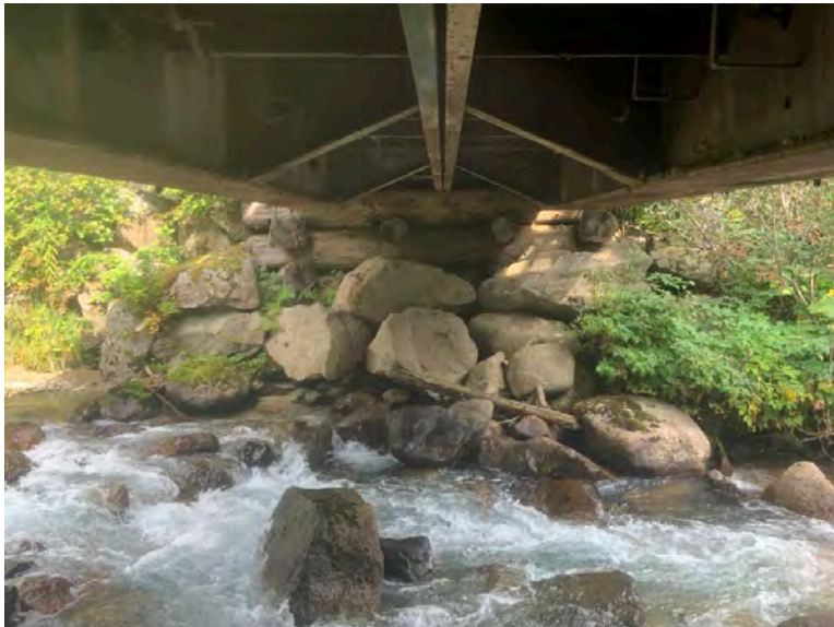
Left Bank Abutment when facing downstream
