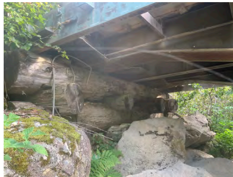
Left Bank Abutment when facing downstream
