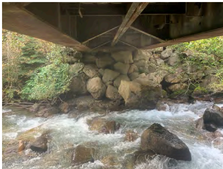
Right Bank Abutment when facing downstream
